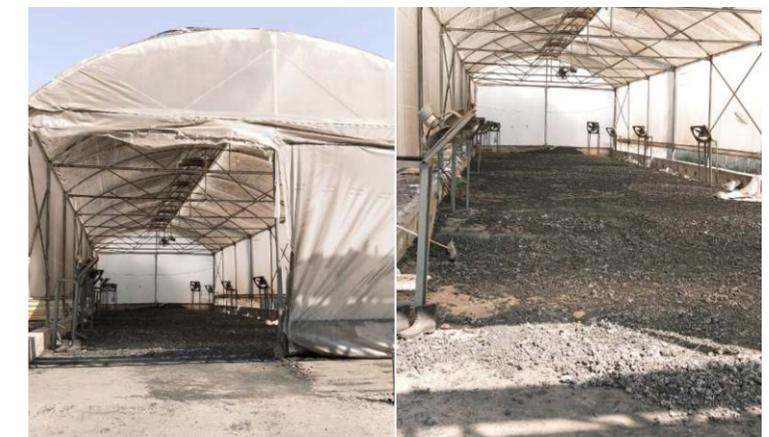
**The initial moisture content of the wet sludge was 82%, however on the fourth day the final moisture content of the sludge was reduced to just 20%.**
